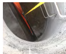
1) Place hose in jaws 2) Close Jaws around hose 3) Lower the guide into place 4) Pull rope and release hose and nozzle
