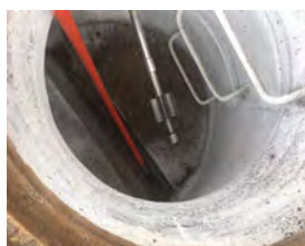
1) Place hose in jaws 2) Close Jaws around hose 3) Lower the guide into place 4) Pull rope and release hose and nozzle
